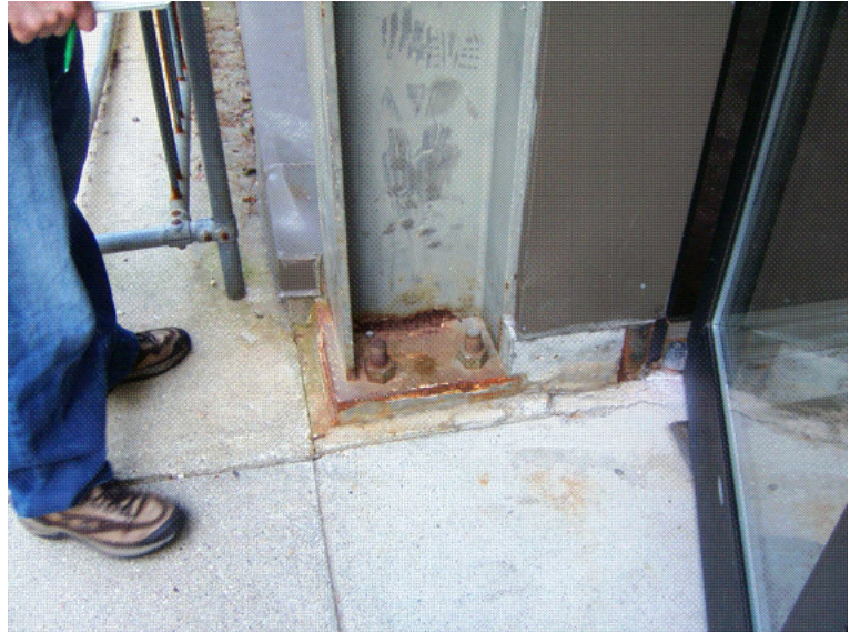
Column bases at main entrance
