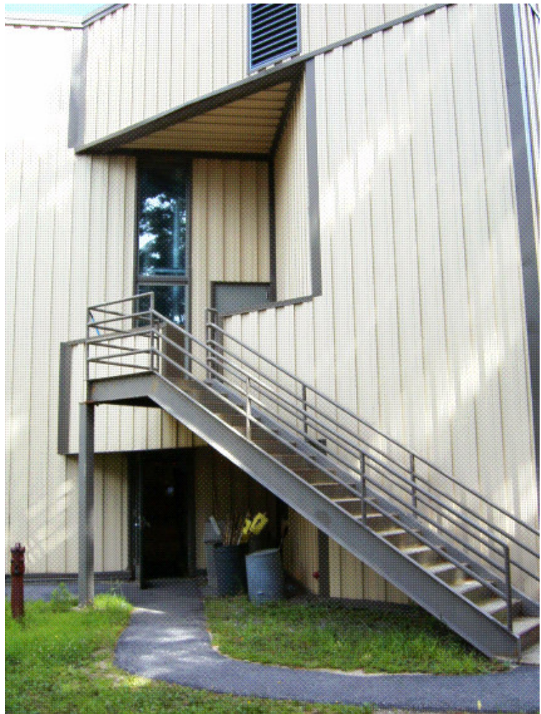
Egress stair at South elevation
